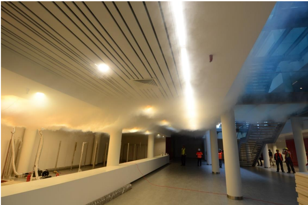
Fig. 5 Hot smoke test in an atrium space. Performance of the system is hindered by the lack of smoke channelling screens.
